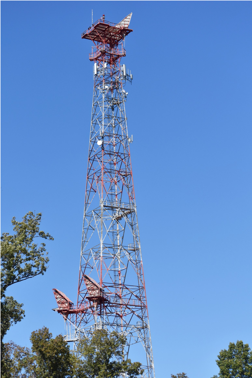
Tower seen from the access of Berry Road.
